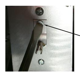
Install the spring over thermostat shaft as shown (arrow). Install the counter-sink screw included with the spring. Tighten the screw, ensuring the spring is positioned as illustrated (arrow).
